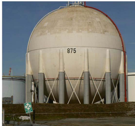
Figure 1-15 : Structures supports de sphères de stockage (TOTAL)
